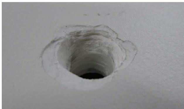
Picture - 1 - Cracks ( \varnothing 8,5 test)
